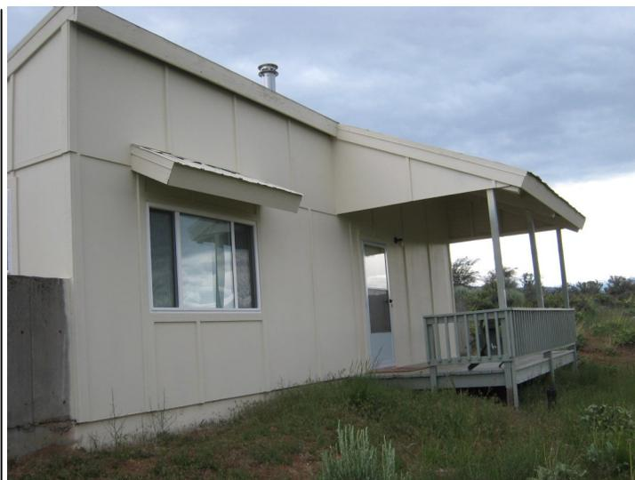
The new Hardi-board siding was chosen because it is so durable with regard to weather and critters. The new windows are more energy efficient and the large window in the main room now has two panels which allow for air flow from screens.
